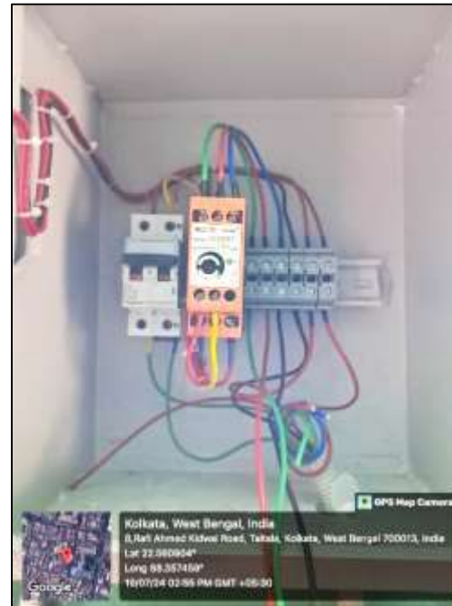
Sensor based auto cut pump motor set in water tank of College building
