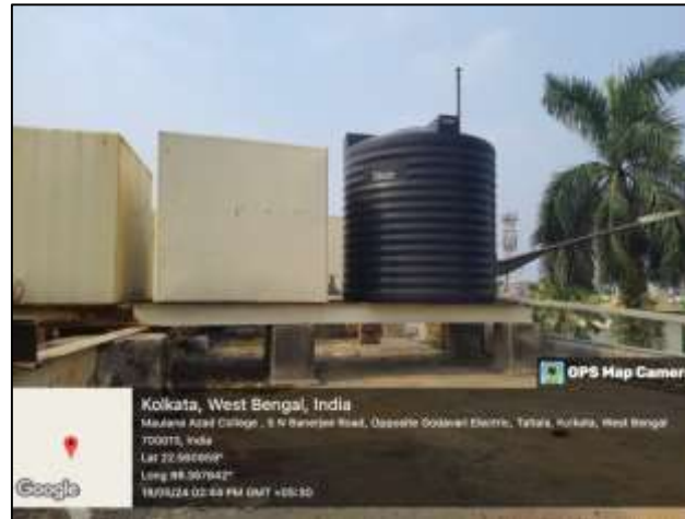
Overhead water tanks in college rooftop
