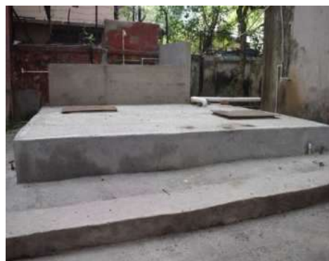
Underground reservoir 1 and 2 at college
