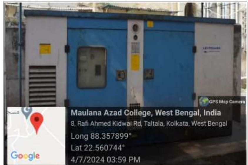
Green Generator Ashok Leyland make 125 KVA capacity
