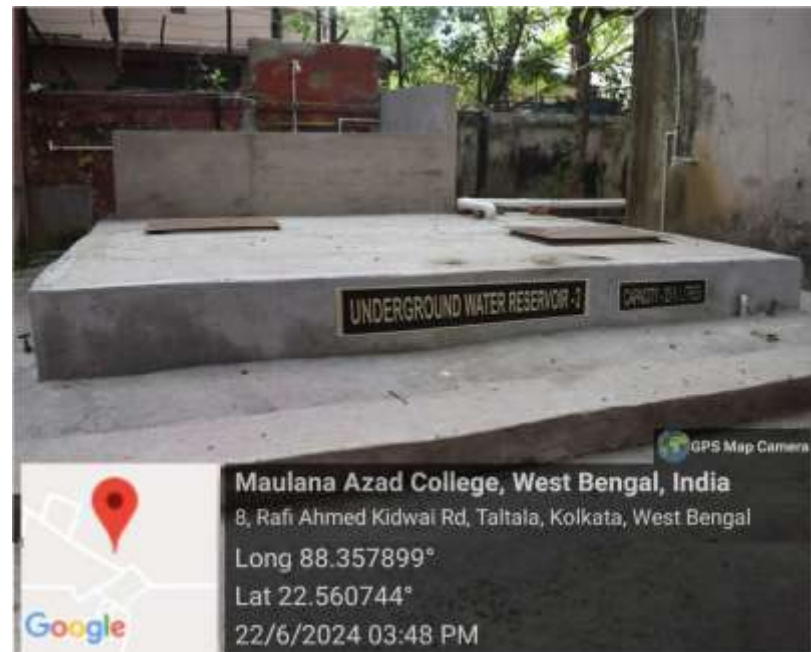
Underground water reservoir 2 (33K ltrs. Capacity)
